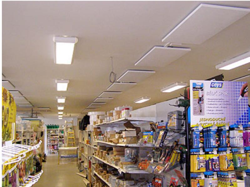
49 ECOSUN 600 U (29.4 kW) panels were installed in three rows in the store. They were basically self-installed by the store. The panels are divided into three sections which can be switched on gradually, depending on the performance requirements. According to the owner of the building, only one section was in operation for the whole 2007/2008 heating season due to the mild winter.
