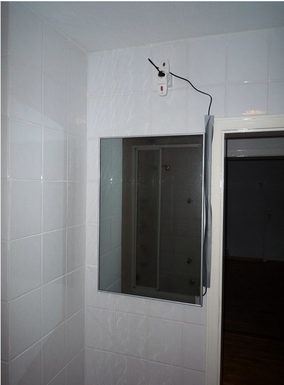
Pic. B3: Bathroom
