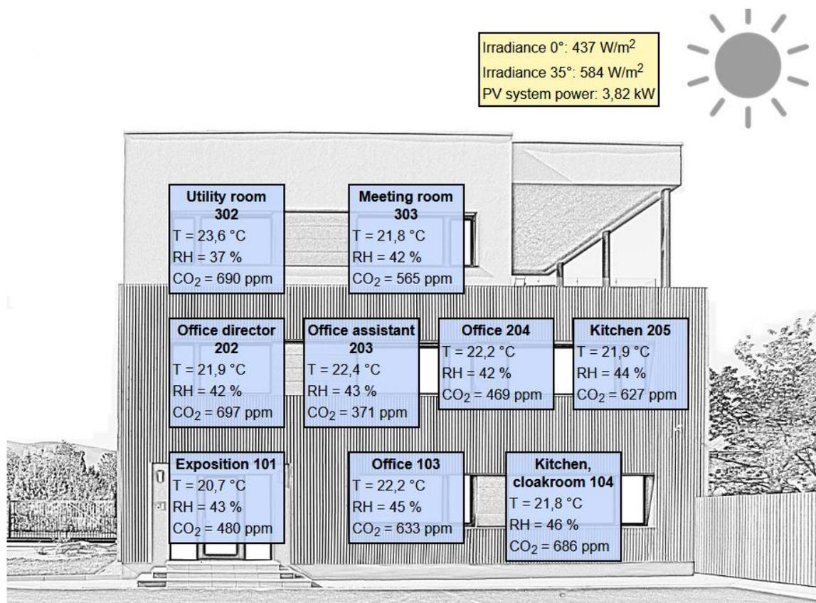
Fig.1 Overview of offices and other rooms with monitored parameters of the indoor environment
