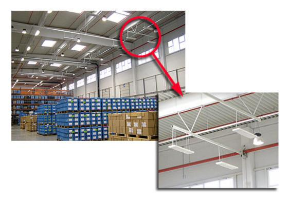
Also, the fact that electric radiant panels are actually a maintenance-free system is a considerable advantage. A gas boiler plant system with an output of 0,5MW is already a source of medium air pollution, the gas equipment is subject to regular examinations and checks, and regular measurements of emissions of the combustion products of the sources of heat (boilers) are needed. There is no such extra expenditure when ECOSUN electric radiant panels are used.
