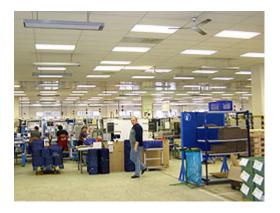
The budget estimate for the setting up of heating with ECOSUN radiant panels was less than half compared to that for competing systems with a gas boiler plant and warm-water or warm-air heating. Also, the costs of the operation of radiant electric panels are about 1/3 lower than when gas heating is used.
