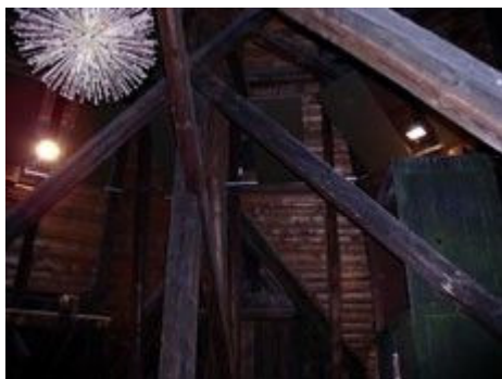
attic Jindrisska Tower
